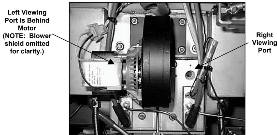
The air/gas mixture is properly adjusted when the burner manifold pressure is in accordance with the applicable table on page 5-8 and the burners display a bright orange-red glow. If a blue flame is observed, or if there are dark spots on a burner face, the air/gas mixture requires adjustment.
