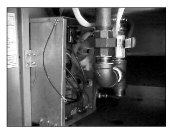
5. Replace the component box cover, being sure to reconnect the ground wire. Replace any drain plumbing components that were removed and reconnect the cooker to the electrical power supply.
