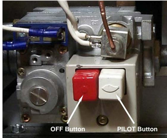
2. Place a flame near the pilot assembly, push and hold the PILOT (white) button in, light the pilot, and continue to depress the button for at least 60 seconds after the pilot lights. Failure to hold the button in long enough will cause the pilot to go out when the button is released. If the pilot goes out when the button is released, wait at least 5 minutes then repeat this step.
