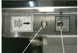
Filter pump reset switch
