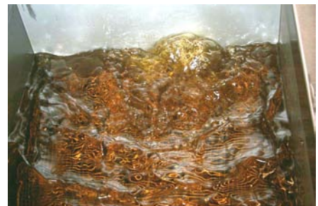
Air bubbles from the Oil Return Line
