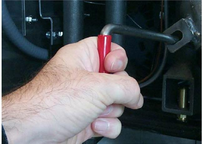
Pull the red handle to open the drain valve.
