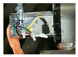
Blower junction box wiring. Mark wire locations before disconnecting each wire.
