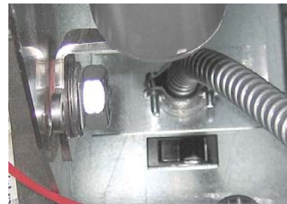
Figure 14 (Rear view of Control Box)
