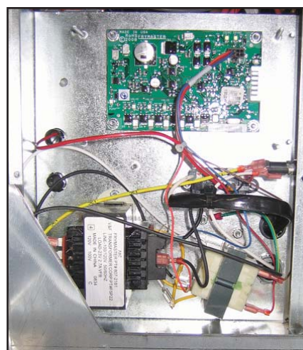
ATO box interior, with LON gateway removed to expose ATO board.
