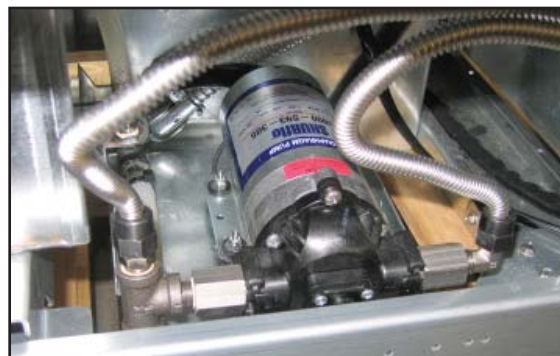
The pump that moves oil from the reservoir to the frypots is visible above.
