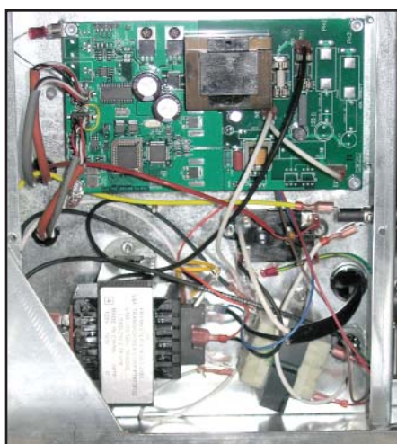
ATO box interior, with LON gateway still installed.
