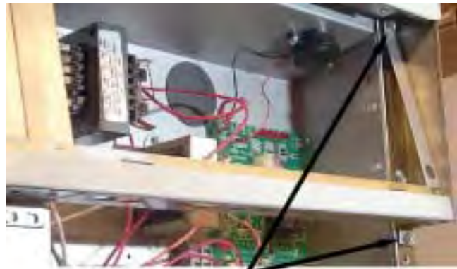
Screws securing control panel frame
