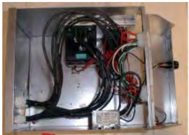
Mark each wire for re-assembly, then remove all wiring connected to the contactor(s) to be replaced.
