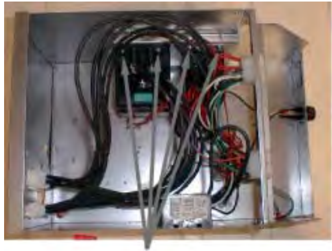
Contactor mounting screws
