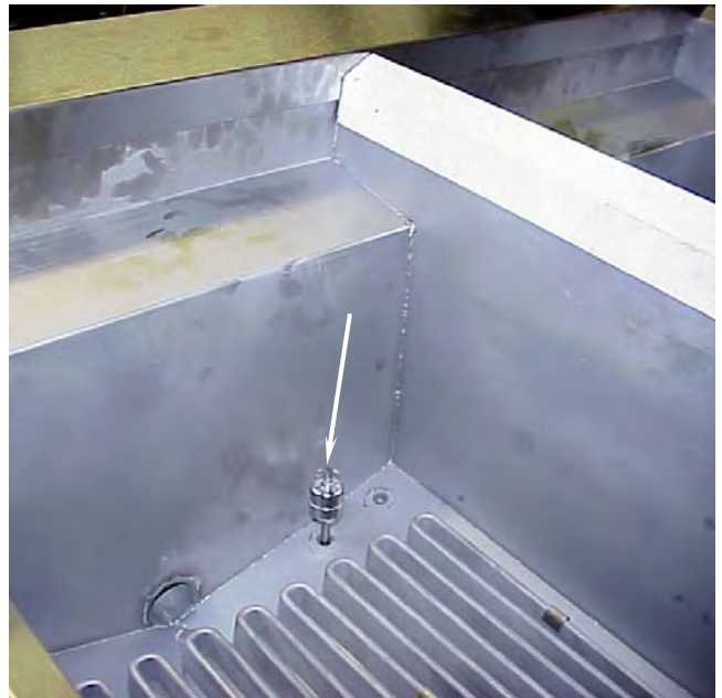
Float safety switch location.
