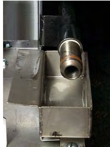
Proper drip pan placement.
