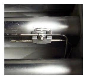
Typical high-limit/sensor probe locations and mounting hardware.
