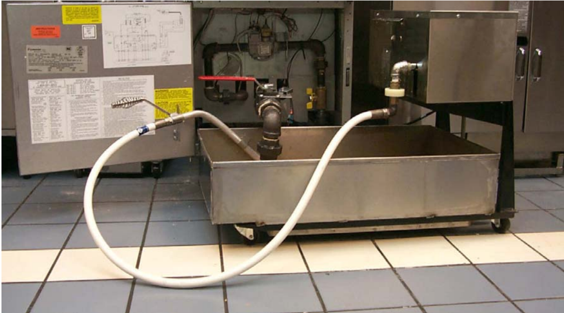
PF95LP portable filter positioned correctly next to fryer drain valve, with rear casters locked in place.
