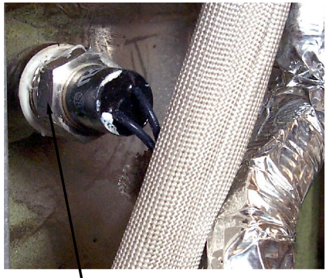
Place wrench here when removing and installing high-limit.
