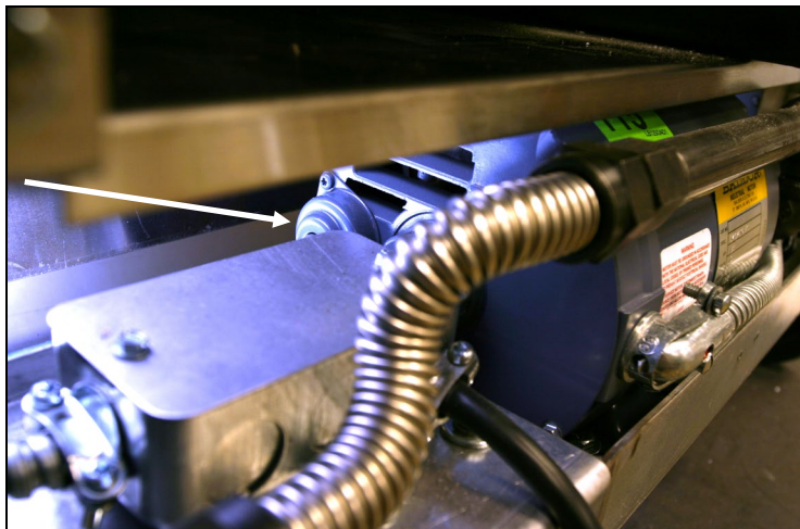
Filter Pump Reset Switch (Arrow)
