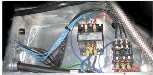
Left and right views of contactor box components.
