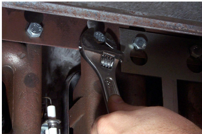
Loosening burner bolts prior to burner removal.
