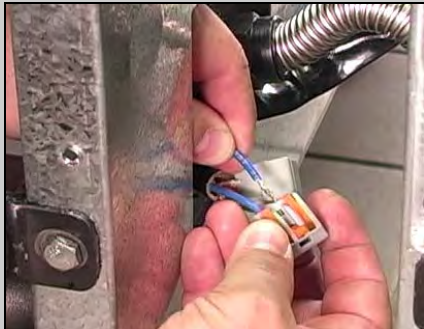
Figure 3: Connecting drain safety wiring.
