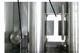
Low-water float switch, Temperature probe
