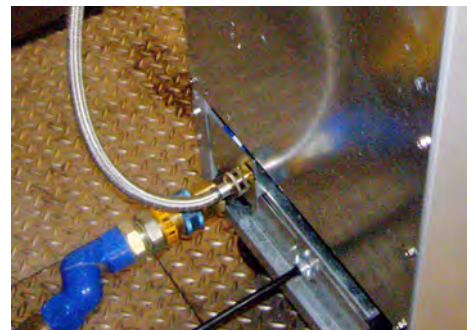
Gas. Water Connections
