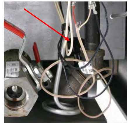
Insert match or taper through this hole to light pilot.
