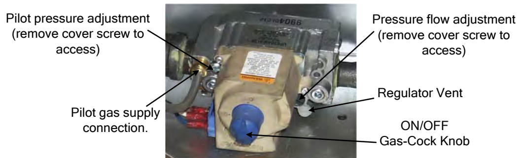
Typical non-CE gas valve for electronic-ignition equipped fryers.
