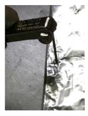
**Fig. 11, 12:** Find the set screws under the foil insulation and push through with an allen wrench.
