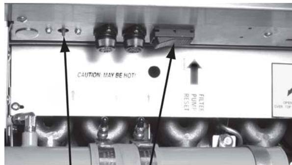
High-limit Reset Switch Manual Filter Override Switch
