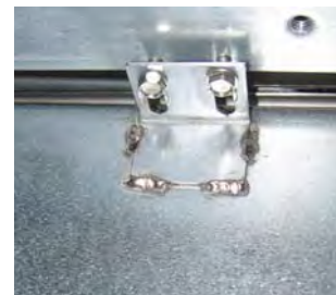
Figure 5: Attach the melting unit to the rails on both sides.
