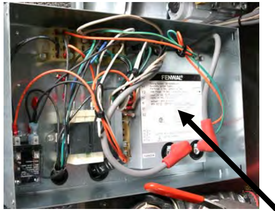
Module located in box below cookpot.
