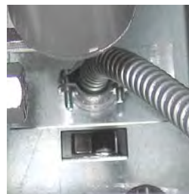
Figure 14 (Rear view of Control Box)
