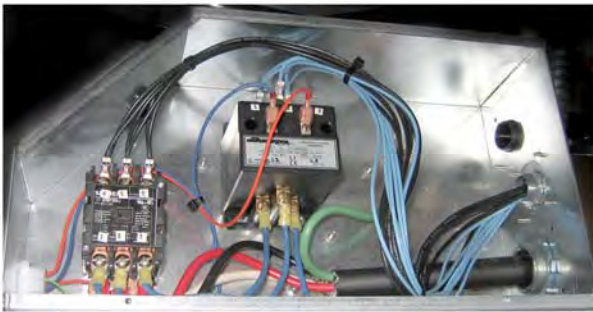
Left and right views of mechanical contactor box components.
