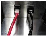
**Figure 2:** The translator connects to the primary holding cabinet with RJ12 cable (right). The secondary cabinet, if present, is connected with CAT 5 cable (left). The primary cabinet must be larger or equal in size to the secondary cabinet.
