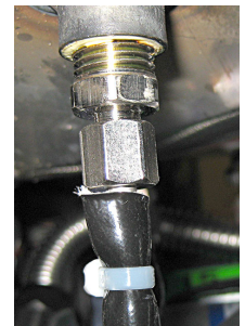
Figure 8 Temperature Probe – Lower View
