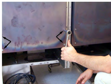
Removing bolts (arrows) securing flue to frypot.
