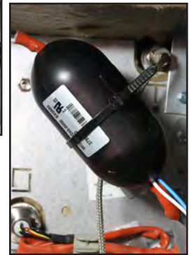
The OIB probe must be regularly cleaned.
