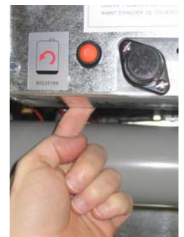
Figure 9 Resetting control power on an electric.
