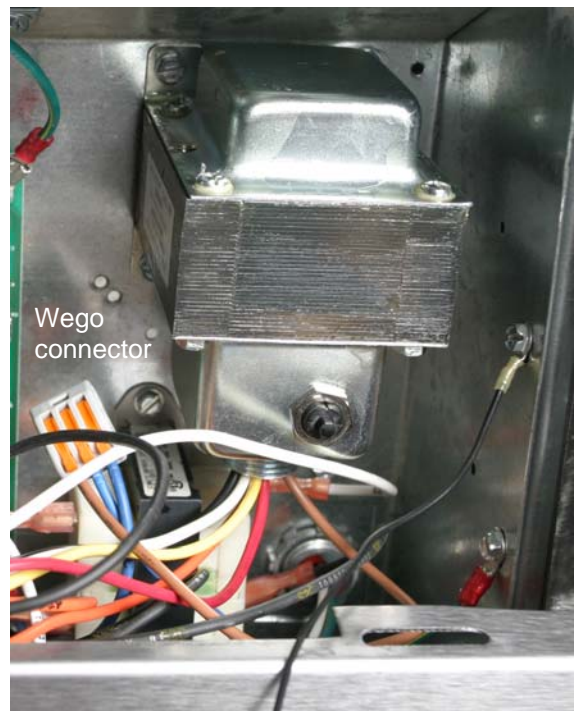
Figure 4: Position the 24-volt transformer as shown. A wiring diagram and an annotated wiring guide are provided on the back.
